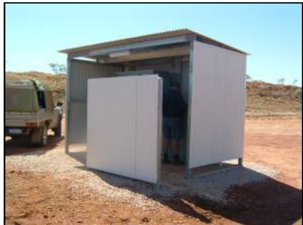
A new shade wall was added to the front and back of the original bus shelter to reduce the temperature inside which was rising to 50C and above over summer, with potentially harmful impacts on the life of the batteries
