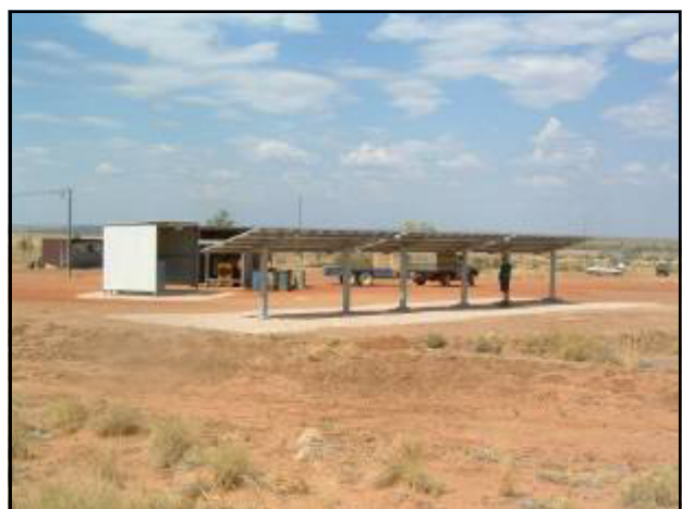
The Mingalkala RE system with 'Bus Shelter' housing for the Bushlight enclosure.
