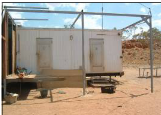
New roofing was since installed to protect some of the transportables from the harsh summer sun.
