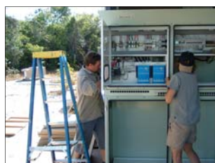
Fitting cables at Bawaka, Top End, NT
