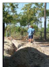
Laying cable at Chuula, Cape York, Qld
