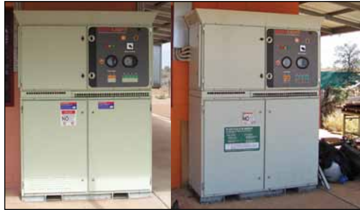
The first Bushlight renewable energy system installed in Dec 2003 at Corkwood Bore in Central Australia (left) and the same system 8 years later (right) after an annual scheduled service
