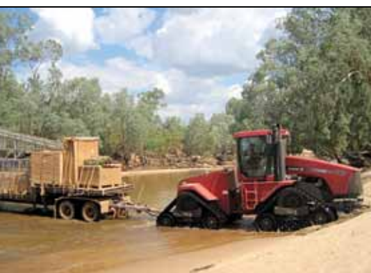
The 4WD tractor getting components across the Mann River in time for installation
