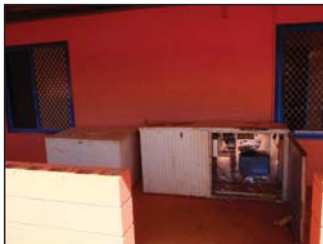
The existing equipment enclosure at 16 Mile was difficult to access
