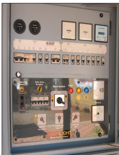
The new escutcheon interface made from durable composite board to prevent peeling
