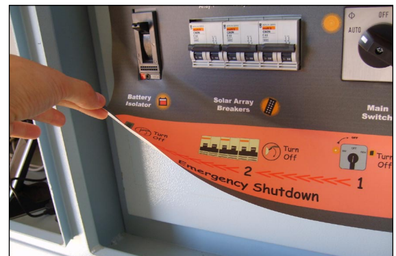
All previous vinyl decals are being replaced by aluminium composite board
