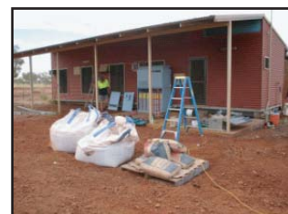
Household system installation underway, Jilariya Kimberley
