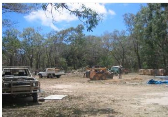
Preparing the site at Moojeeba
