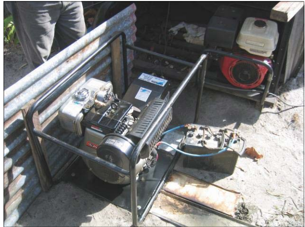
Diesel and petrol generation provided power 6 hours a day pre-Bushlight
