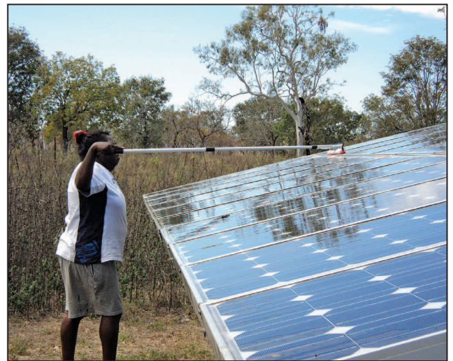
Selma Hoosan cleaning the solar panels during Bushlight RE System Maintenance training at Sandridge in June 2012
