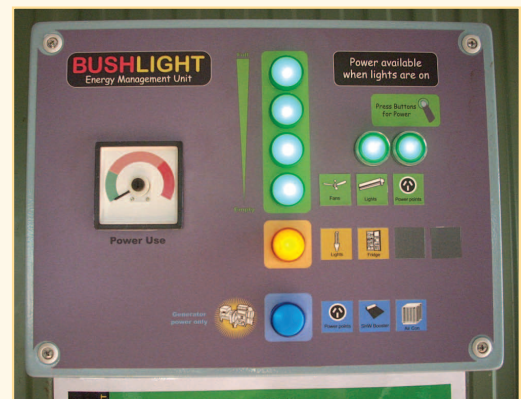
The Bushlight Energy Management Unit user interface helps household residents manage their energy consumption
