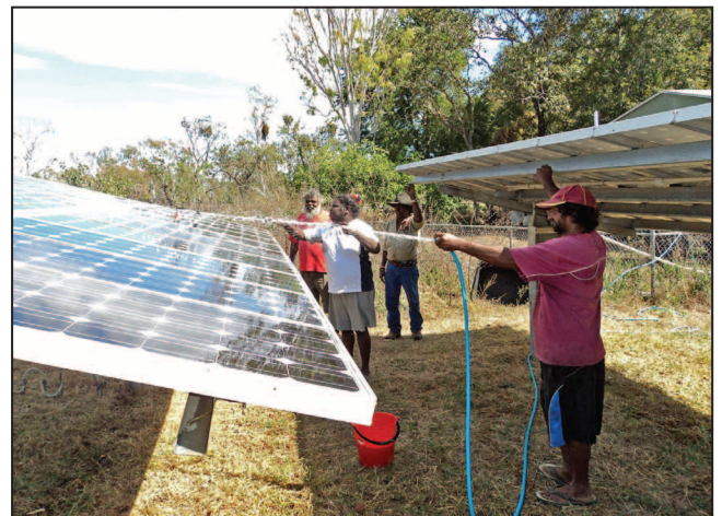
Selma Hoosan and William Coolwell cleaning array panels at Sandridge community.
