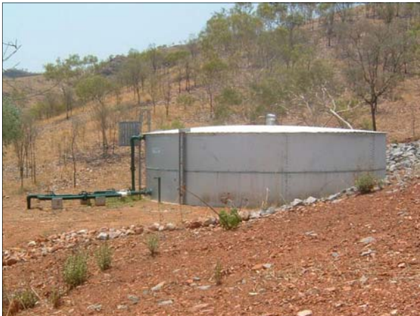
New water tank and pipe work
