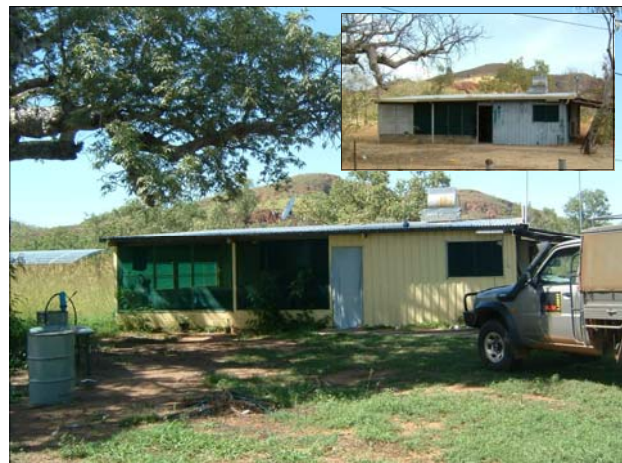
House 3 after renovations (insert shows condition of house when Bushlight first visited the community)
