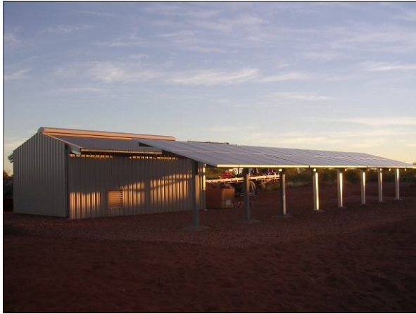
Blue Bush RE System being installed, May 2006
