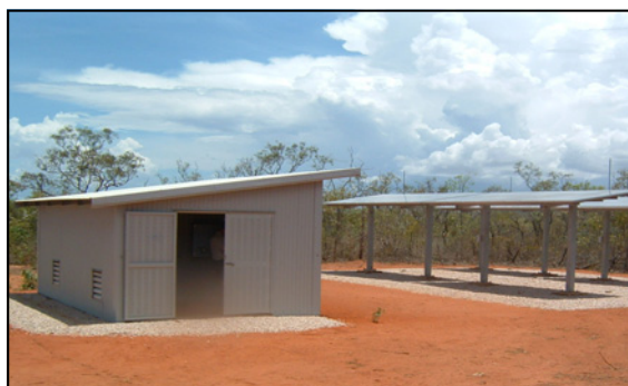
The Bushlight shed and arrays at Munget
