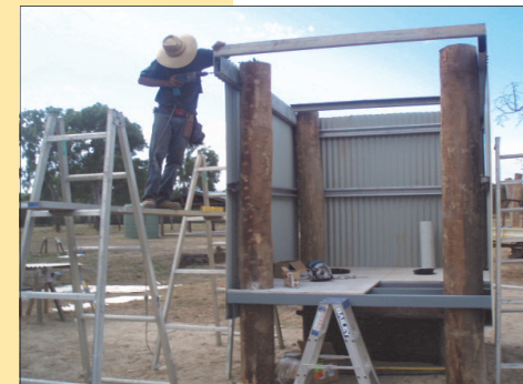
Constructing the campsite toilet at Port Stewart
