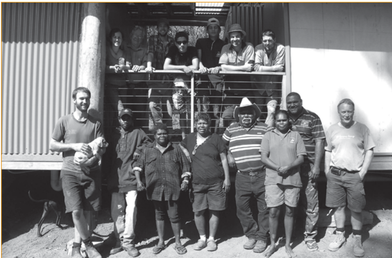
Stakeholders and community participants at newly completed Ranger Base at Shipton's Flat.
