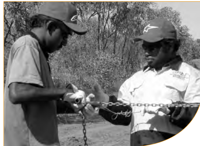
Learners building a fence as part of the Elliott Training Program.
