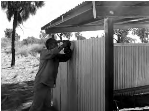
CAT staff build a shelter for Patji Outstation.
