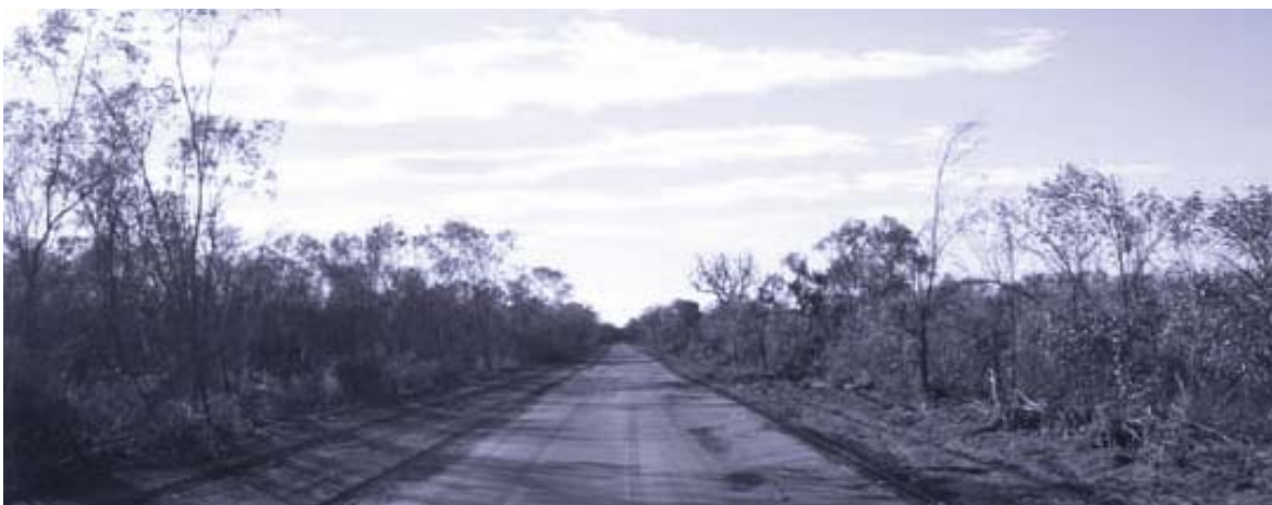
Figure B7.9: Type 1 flat-graded formation access road
