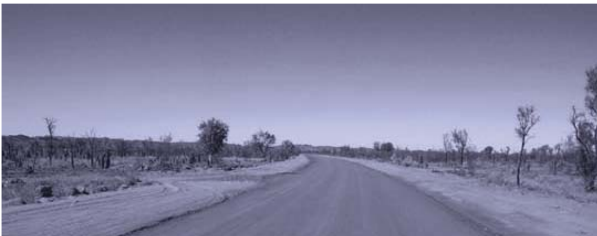
Figure B7.4: Gravel formation access road
