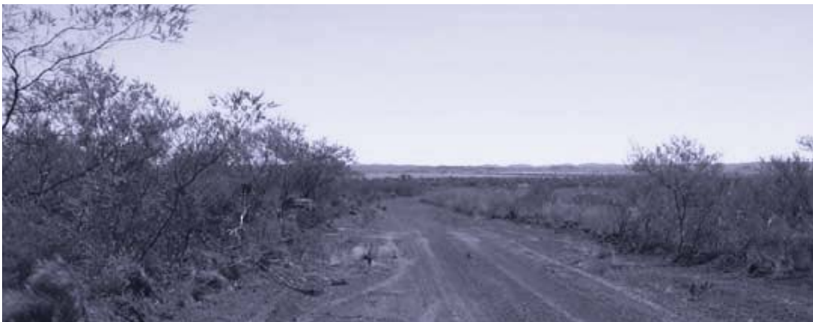
Figure B7.7: Type 2 — formed formation access road
